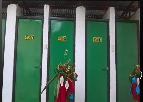
Reinforced steel doors, new roofing
