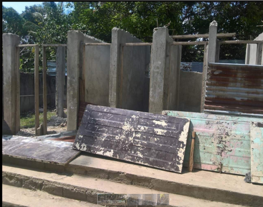
Aftermath of major earthquake (October 2013)
