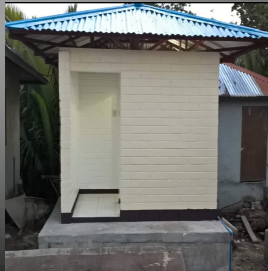
A new bathroom built
